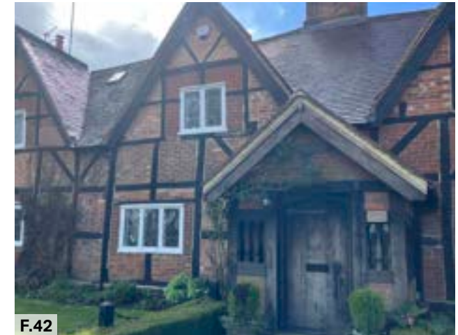
F.42 Figure 42: The Old Hall, a restored 17th Century Hall of local historical importance with red brick, timber frame and gable porch.
