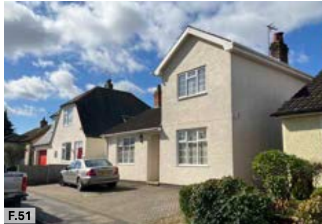
Figure 51: A variety of building heights and roof pitches along North Road, including an uncommonly seen jerkinhead roof.
