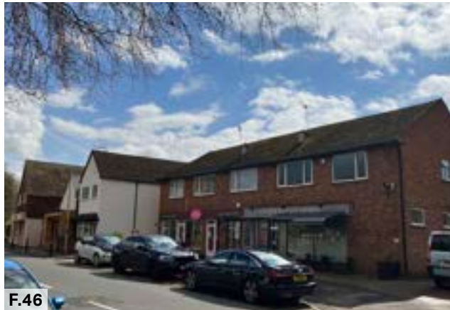
Figure 46: Shop fronts with parking bays and setbacks along High Street within the village core.
