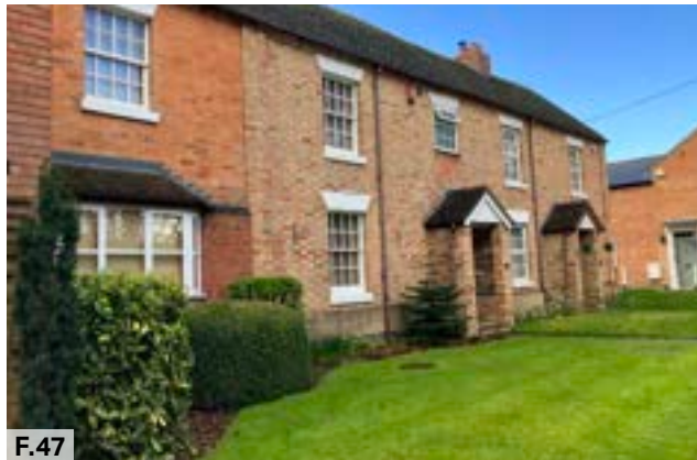
Figure 47: Terraced cottages featuring heritage features such as wooden sash windows with glazing bars, render lintels and weatherboarded dormer porches.
