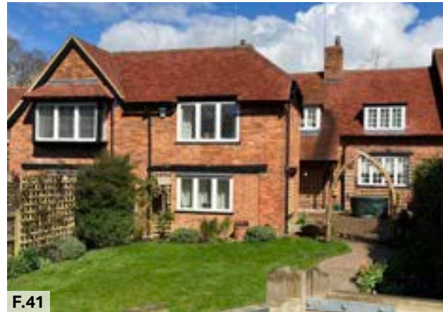
F.41 Figure 41: Restored cottages accessed from courtyards to the rear, underscoring the rural feel of Clifton upon Dunsmore.
