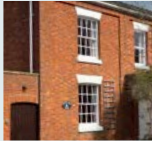
Sash window with glazing bars
