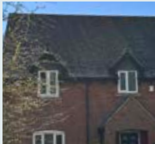
Gable dormer windows
